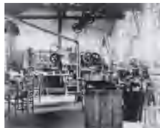
Interior of the factory on Calle Pare Roca, Olot 1925
